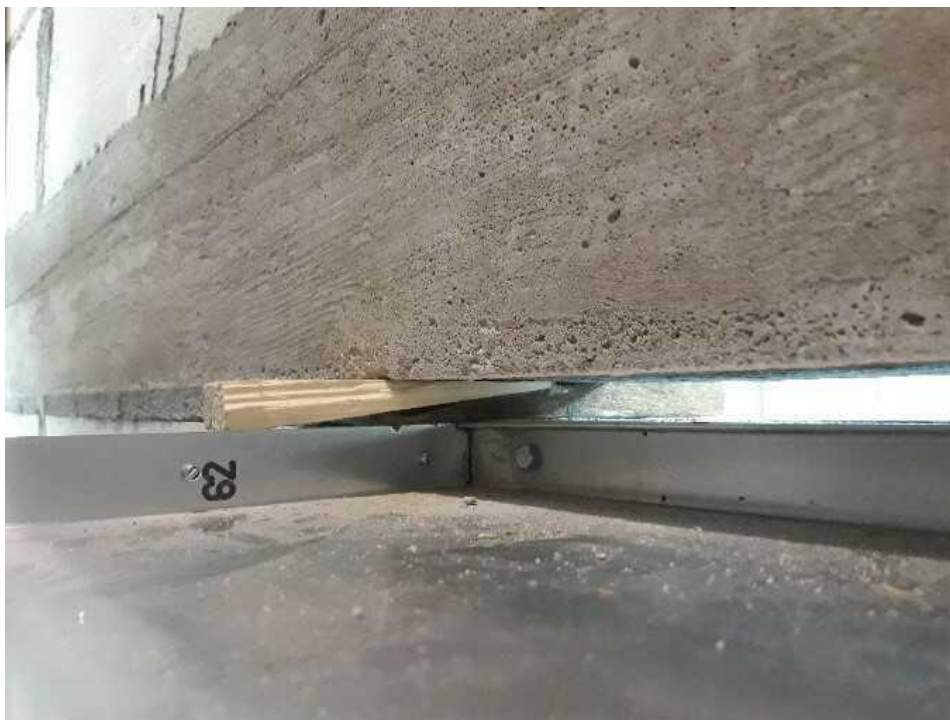
Figure 3. Correct preparation of the damper for installation (using mounting wedge)
