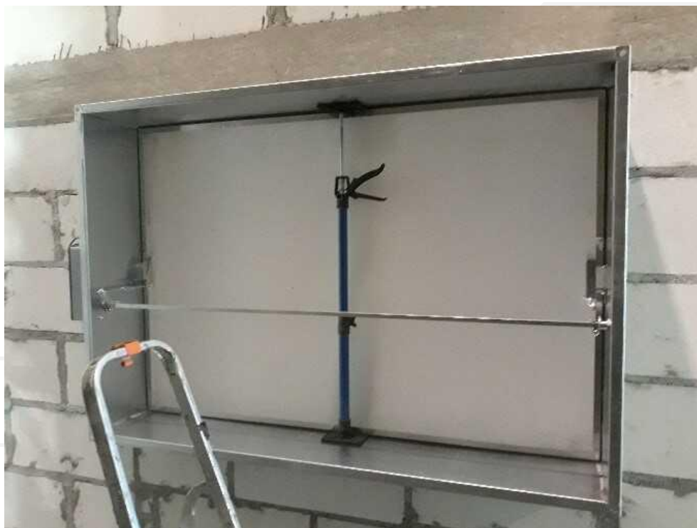
Figure 1. Correct preparation of the damper for installation (using spreader securing the housing)
