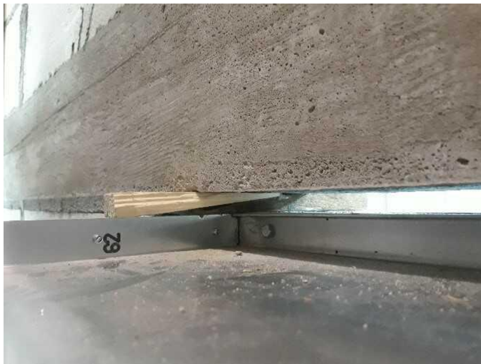
Figure 2. Correct preparation of the damper for installation (using mounting wedge)
